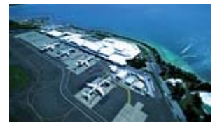
A small boat is identified by this video surveillance system as it approaches an area marked off near an airport's shoreline. Photo courtesy of ObjectVideo
